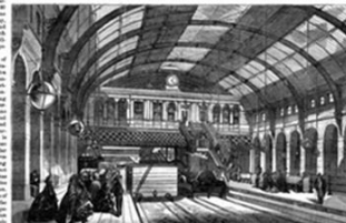
THE LONDON TUNNEL SHOWS IRON GIRDERS.
